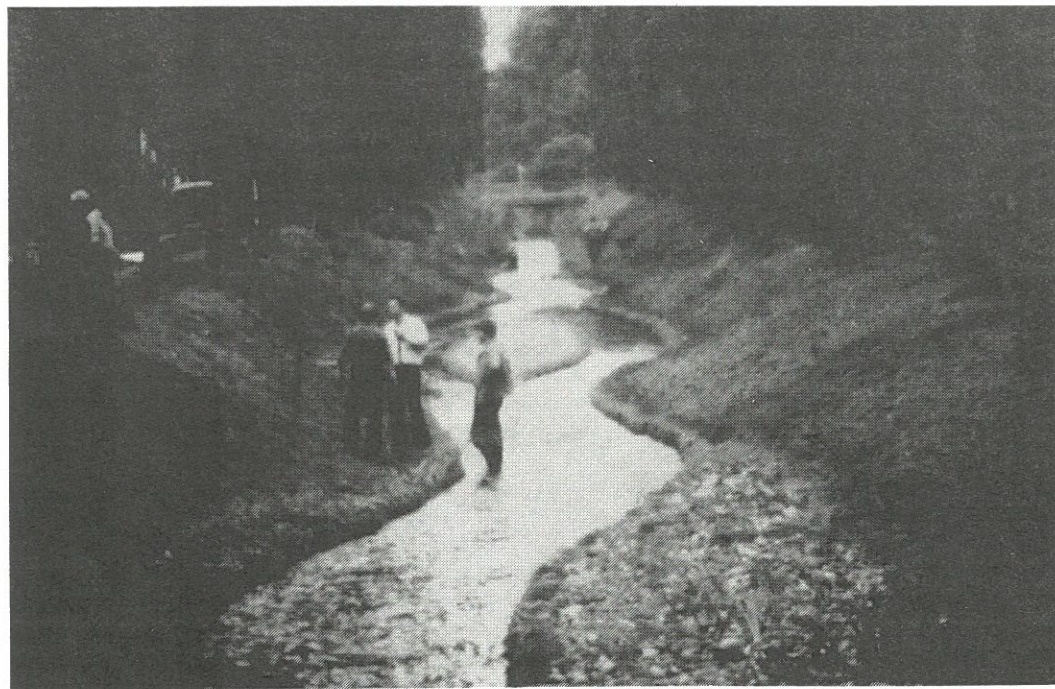
Near complete restoration of a canal in Bavaria, Germany.
