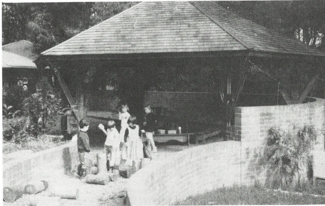
Pagoda adjoining kindergarten buildings at Lorien Novalis School. Architect: David Jacobson.
